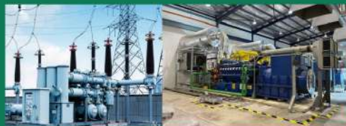
Construction of Biogas Power station for electrical generation
